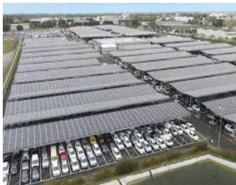
(Charging station for PEVs)
