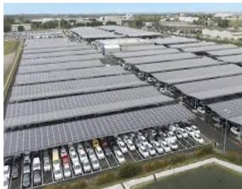
(Charging station for PEVs)
